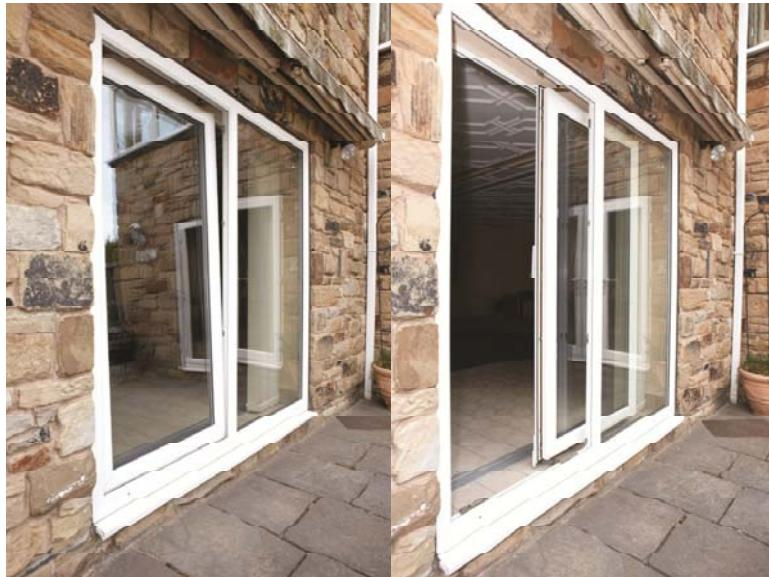
The Tilt & Slide is a premium door solution for spaces that do not allow for inswing doors. The unique sash design tilts and slides parallel to the fixed unit with the touch of a finger. Compression-seal technology contributes to outstanding performance.
